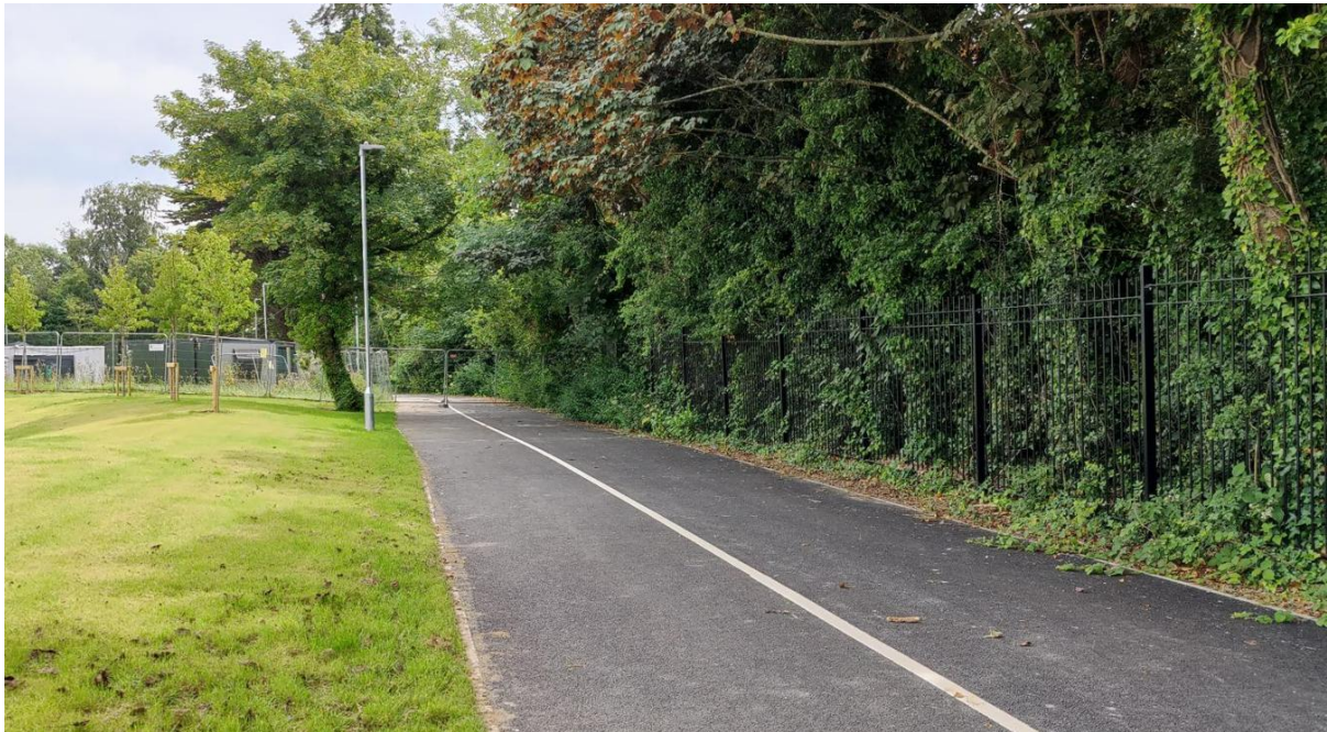
Figure 4-2 Photo showing recently constructed route through St. Joseph's Clonsilla development
